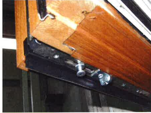
Picture 8 Locking situation casement member 1
