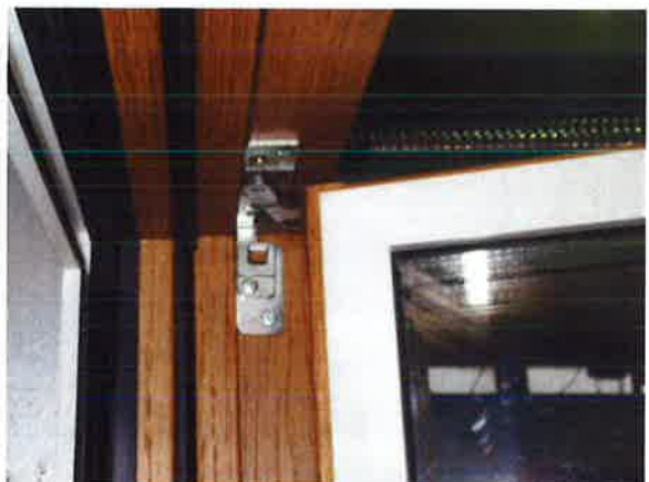
Picture 4 Stay arm bearing, rebate view, turn-tilt leaf
