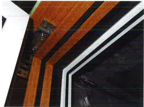
Picture 2 Corner detail frame
