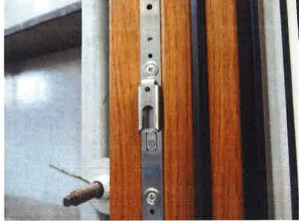
Picture 14 Locking situation frame member 4
