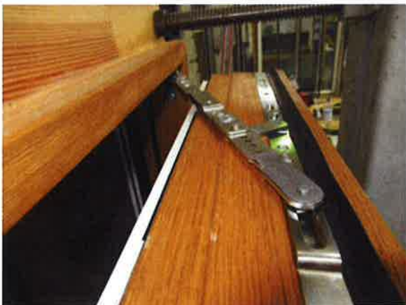
Picture 5 Stay arm bearing, turn-tilt leaf
