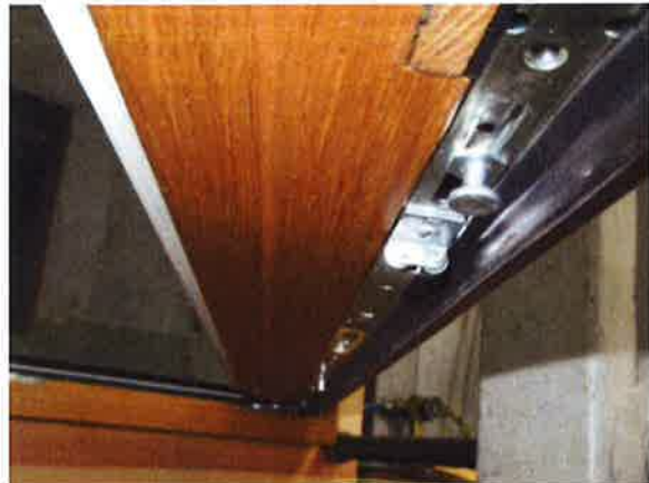
Picture 10 Locking situation casement member 1
