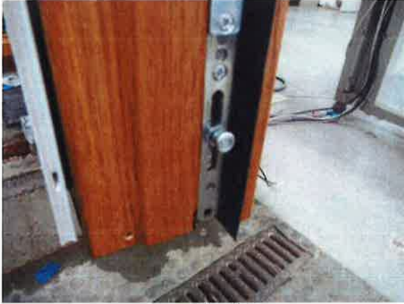
Picture 13 Locking situation casement member 3
